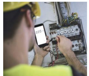
Electric Power Inspection
