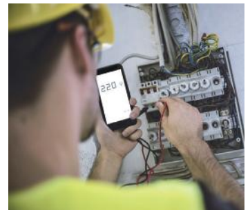
Electric Power Inspection
